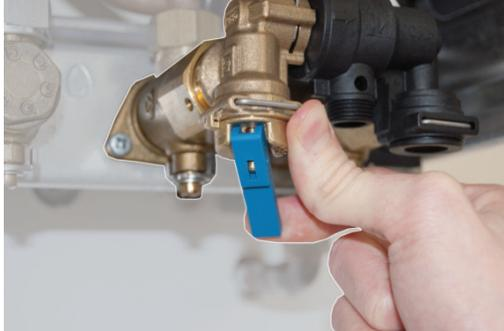
In the case of the keyless filling link, the system is filled using an integral lever. To access the filling link, remove the bottom panel by pulling the catch down and then pulling the panel forward and down to remove.
