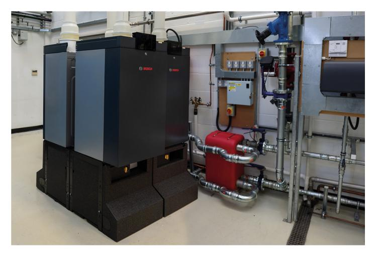
Available in outputs of 50, 65, 85, 100, 125 and 145kW. The Condens 7000 WP can be cascaded in banks of up to 6 boilers per bank providing up to 858.6kW at 50/30 per bank.
