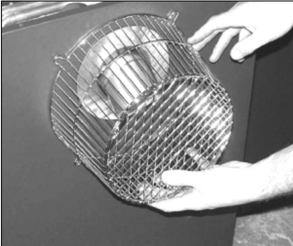
FITTING THE FLUE GUARD
